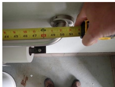
Figure 604.5.1 Side Wall Grab Bar at Water Closets
