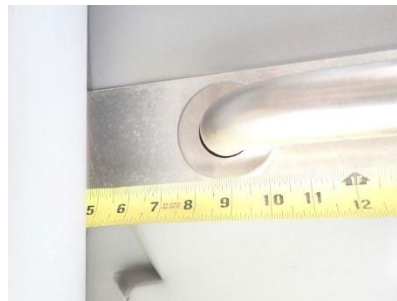
Figure 604.5.2 Rear Wall Grab Bar at Water Closets
