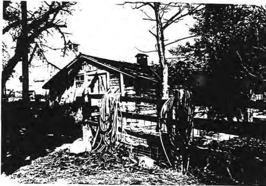
5BL4884 Building 4 Chicken House Front 3/4 to northeast
