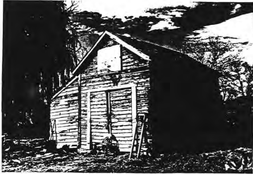
5BL4884 Building 3 Garage Front 3/4 overview to northwest
