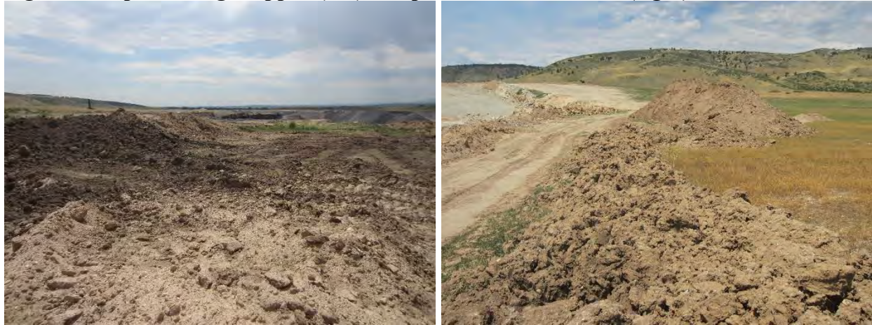
Figure 2: Topsoil being stripped (left) and pushed into windrows (right)
