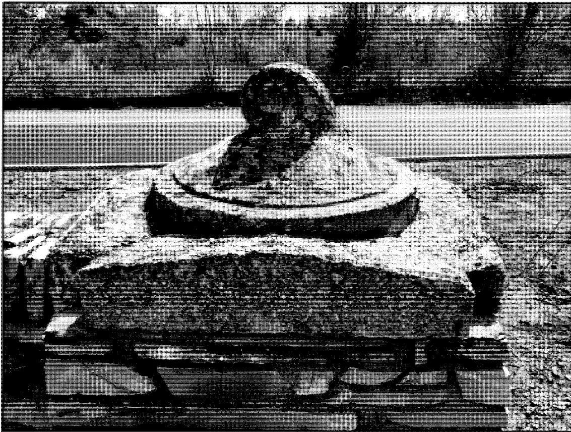
5BL.432, decorative cast concrete element placed on top of end pier of southern gateway pillar, looking south.
