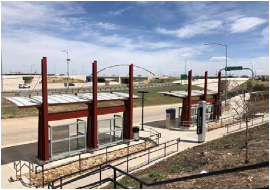
Existing: RTD Station
