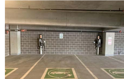
EV Charging Stations
