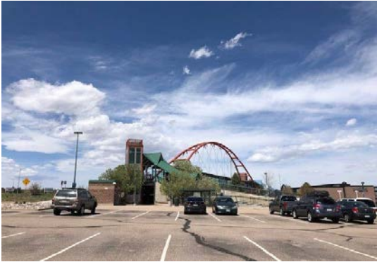
Existing: McCaslin Bridge
