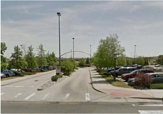
Existing: Center Drive
