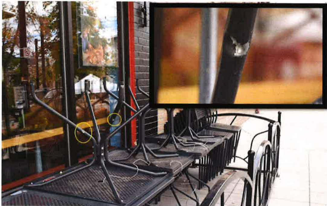
Image taken facing west depicting damage on table legs believed to be from rounds fired during the incident. On the tables and ground investigators found suspected bullet fragments.
