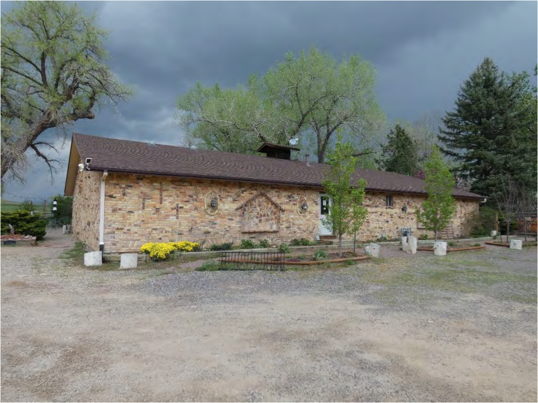
Clubhouse South Elevation May 2021
