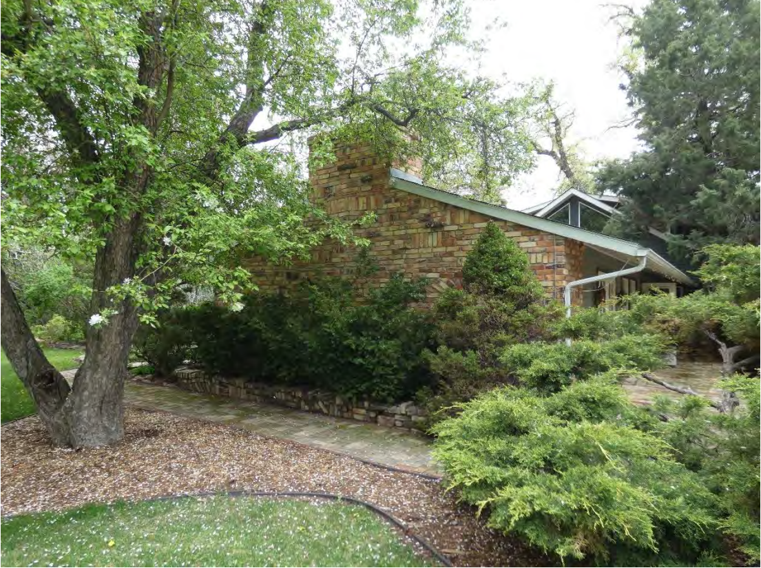
House North Elevation May 2021
