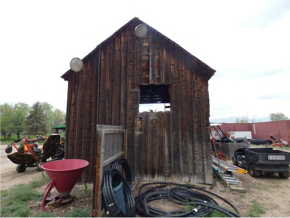
Barn East Elevation May 2021
