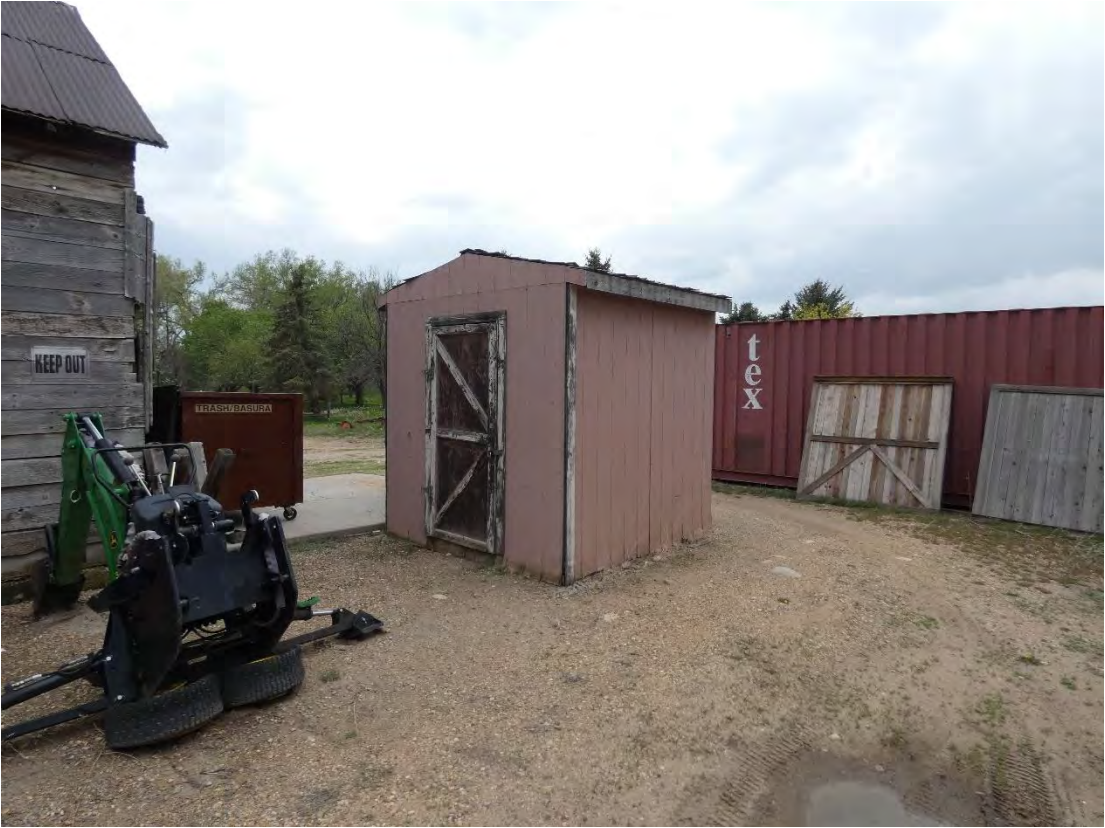
Wood Shingle Shed Northeast May 2021
