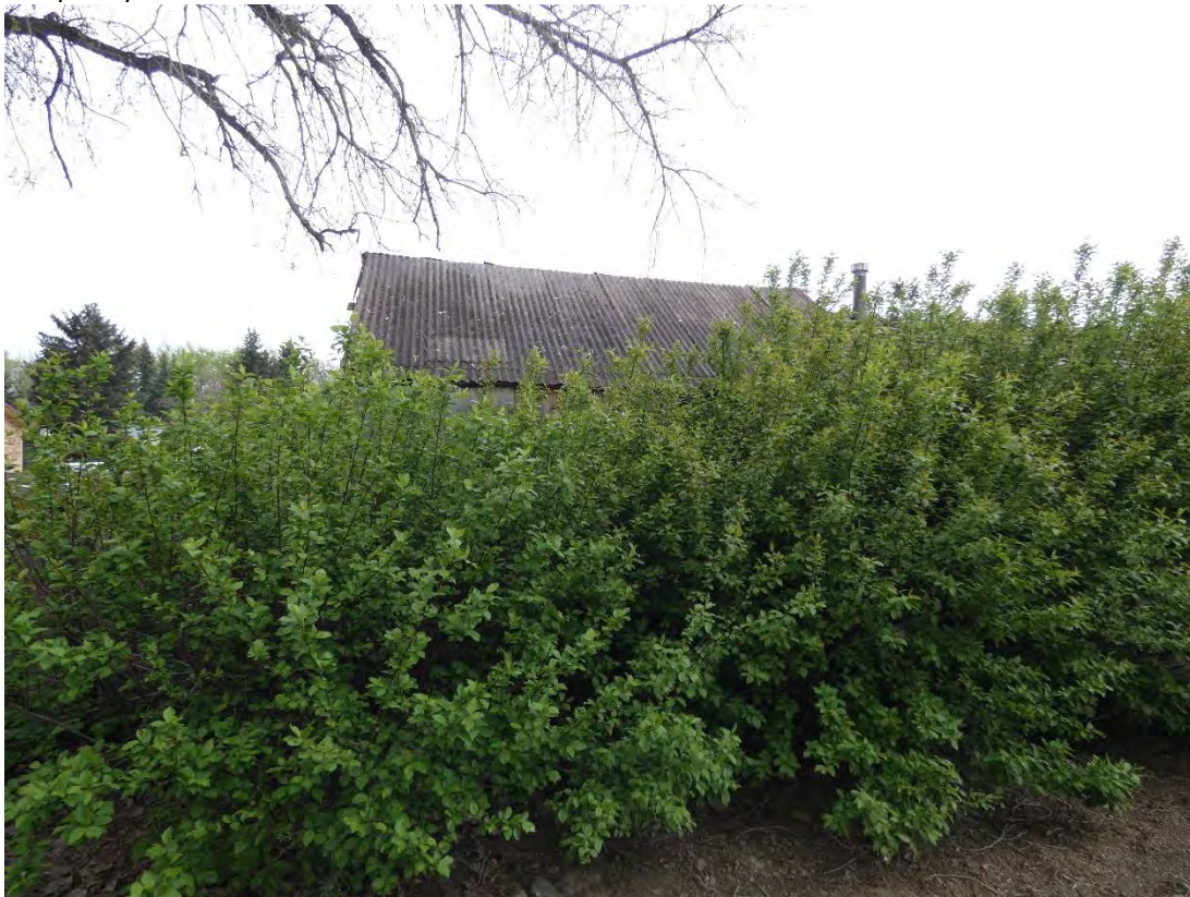
Shed with Corrugated Roof North Elevation May 2021
