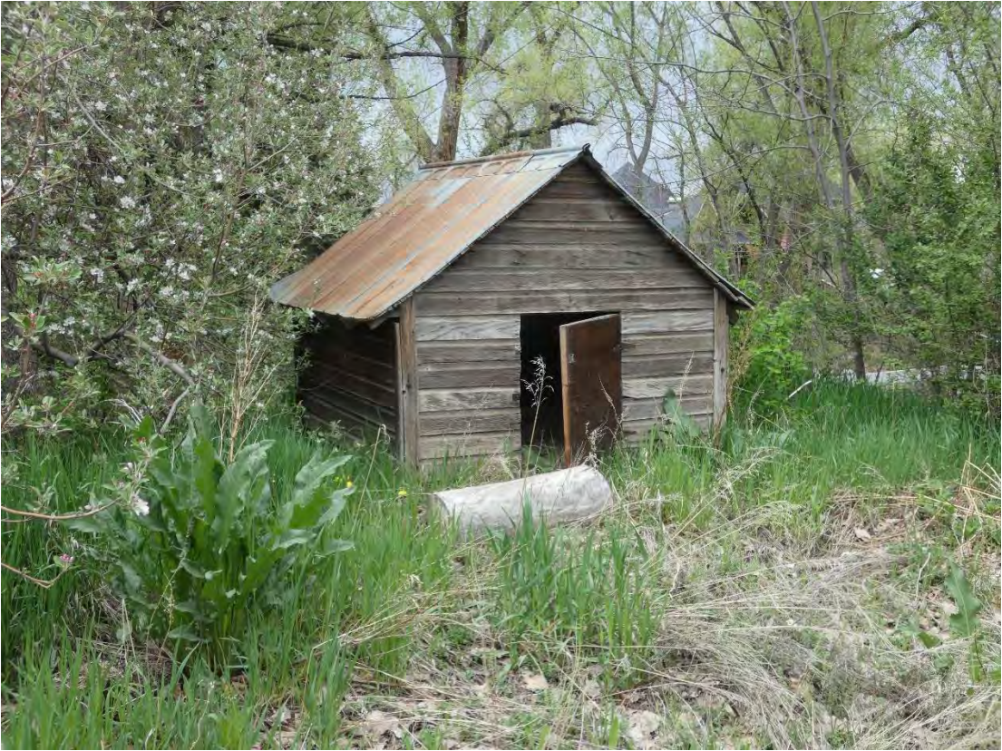
Pig Shed near road May 2021
