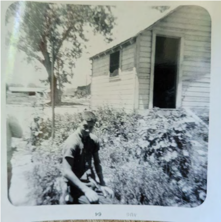
Demolished Structure Person Unkown Circa 1964 Heather Ebel Photo
