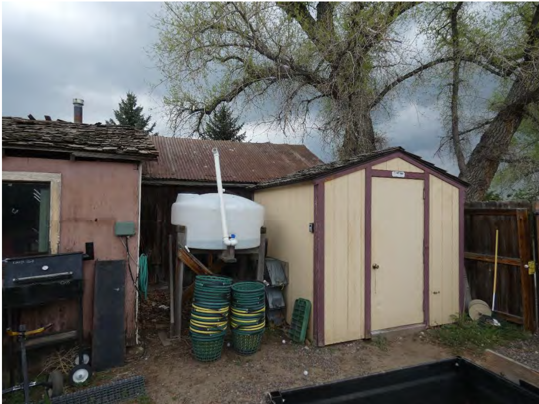
Tan Shed Southwest Elevation May 2021
