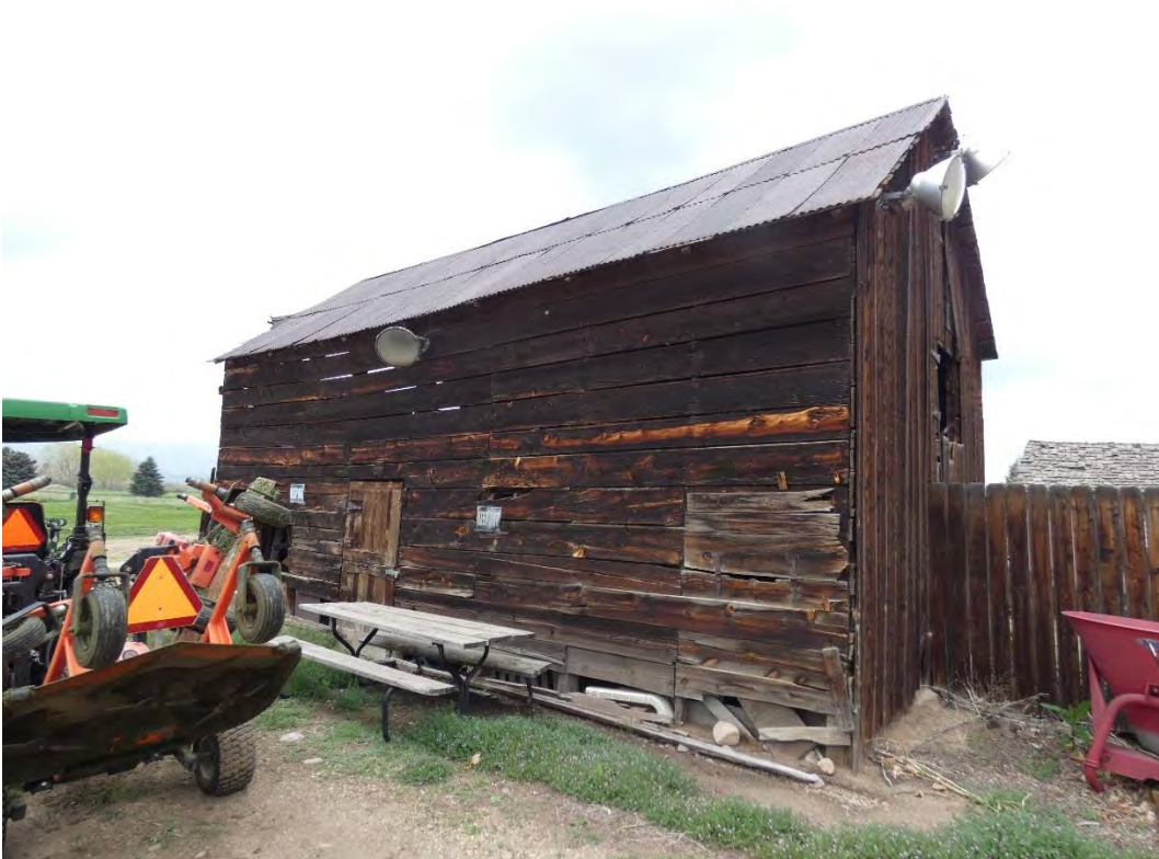
Barn South Elevation May 2021
