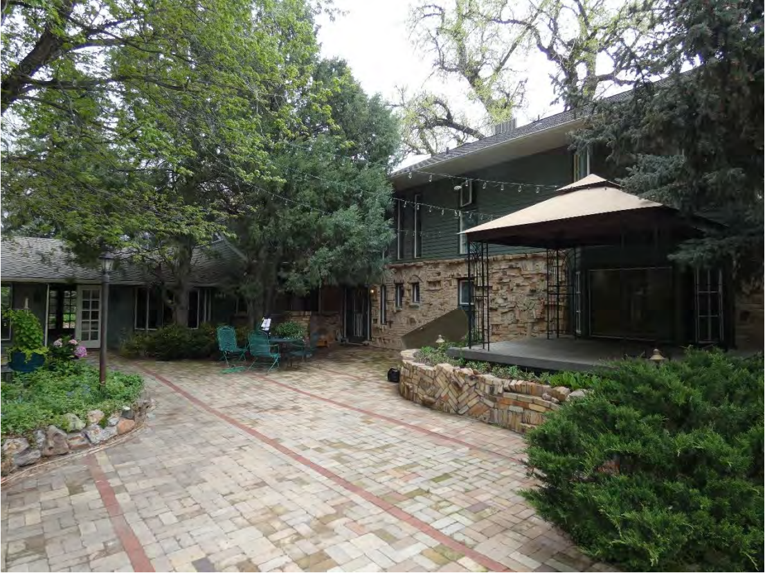
House Northwest Elevation May 2021
