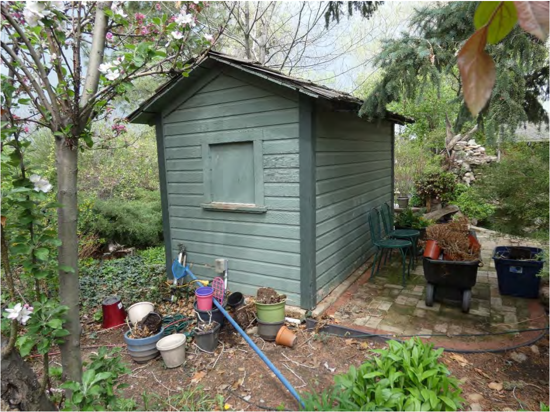
Green Shed Southwest Elevation May 2021
