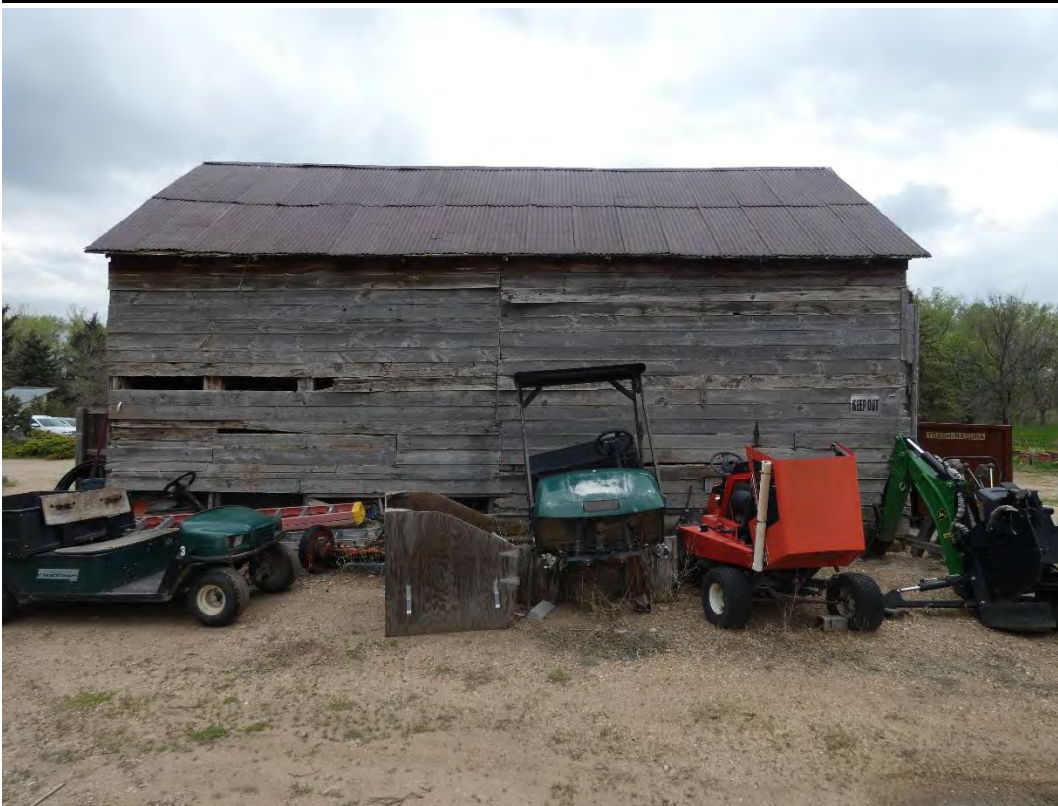
Barn North Elevation May 2021
