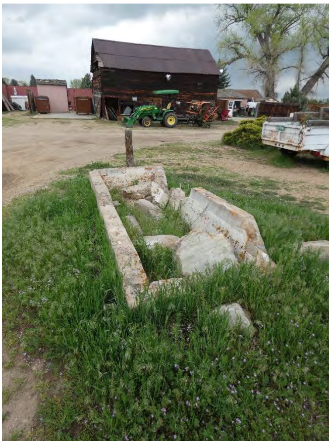
Concrete Trough May 2021
