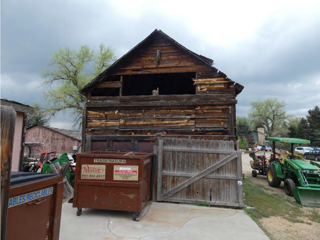
Barn West Elevation May 2021
