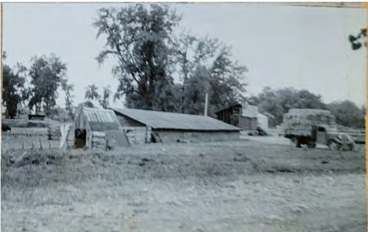
Demolished Structure Circa 1963 Heather Ebel Photo
