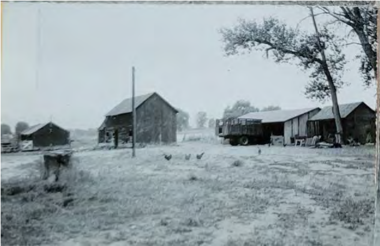
Demolished Structure (Left) Barn (Center), Garage and Shed w/ corrugated Roof (Right) Circa 1963 Heather Ebel Photo
