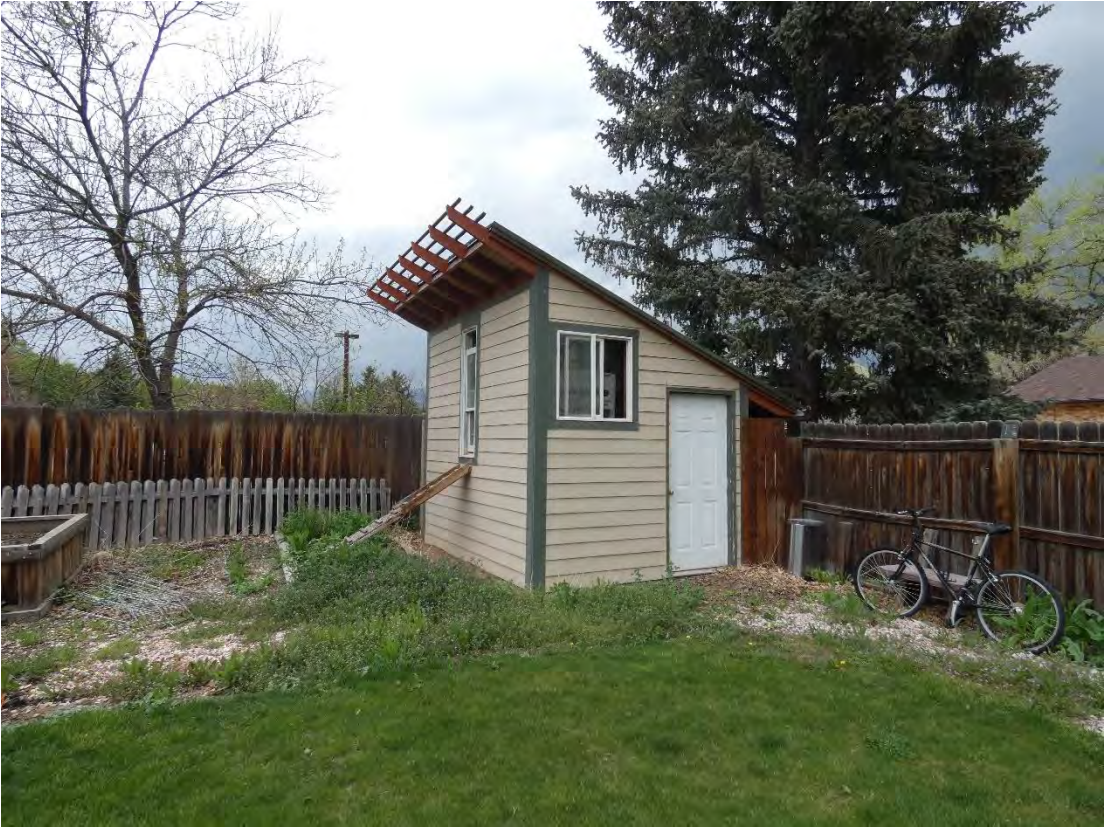
Shed with Shed Roof Southeast Elevation May 2021
