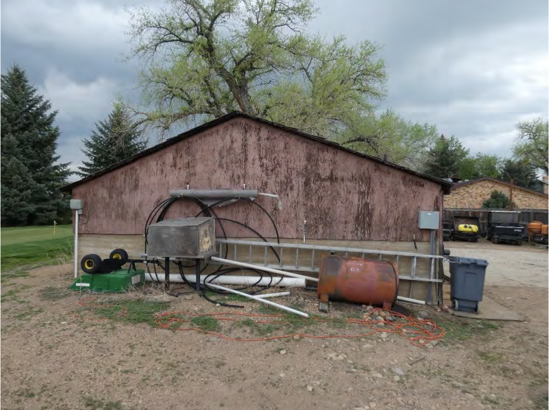
Garage West Elevation May 2021
