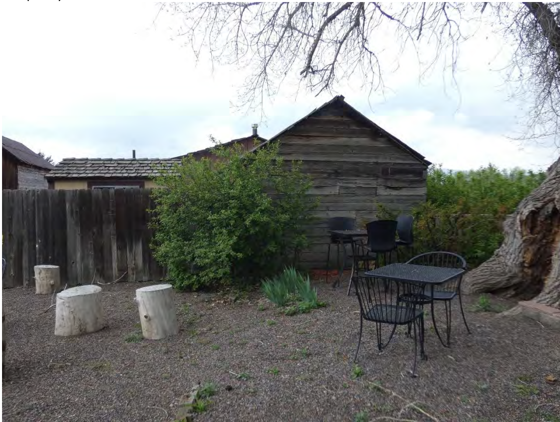
Shed with Corrugated Roof East Elevation May 2021
