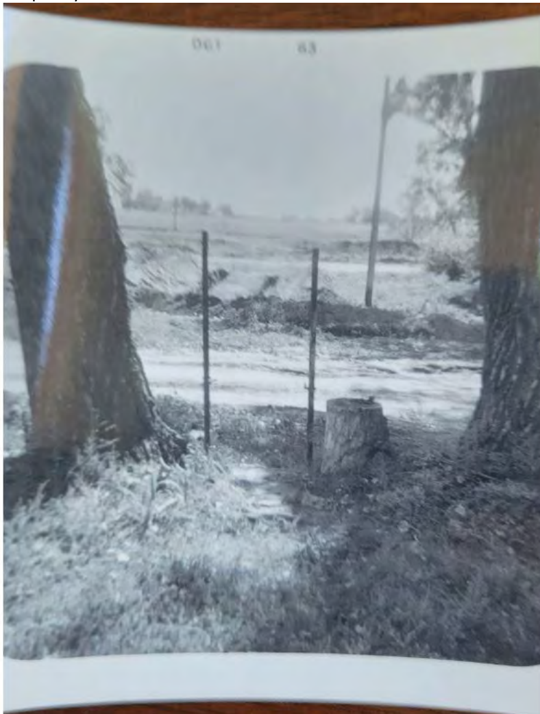
Golf Course under construction Circa 1963 Heather Ebel Photo
