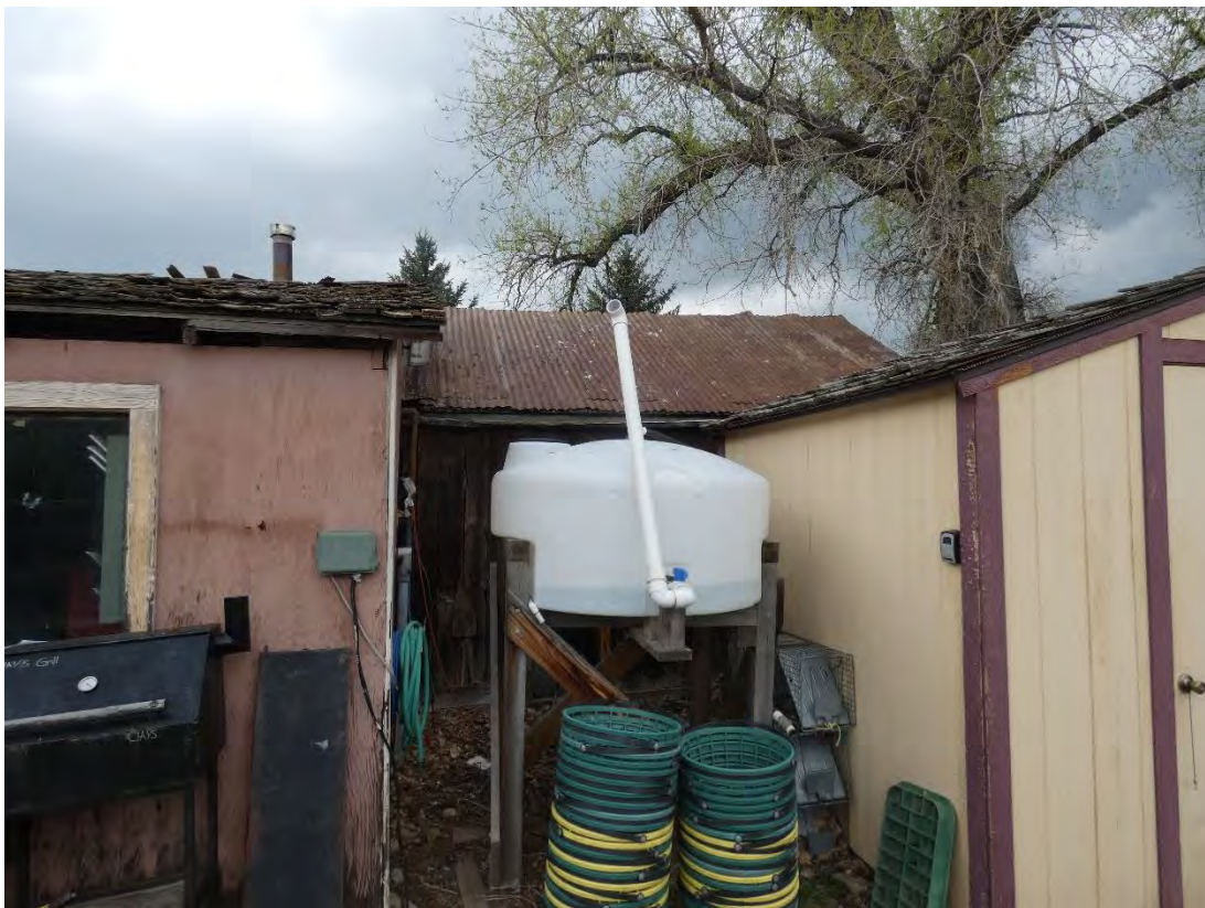
Shed with Corrugated Roof South Elevation May 2021
