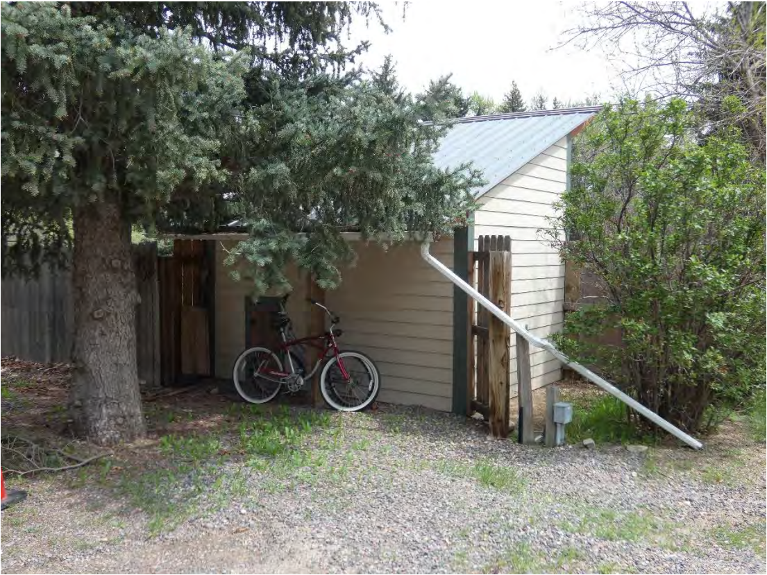
Shed with Shed Roof Northwest Elevation May 2021
