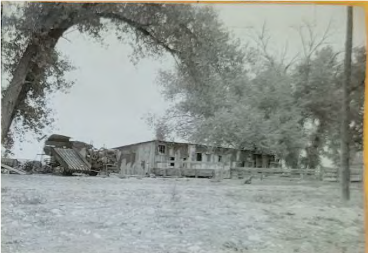
Demolished Structure Circa 1963 Heather Ebel Photo
