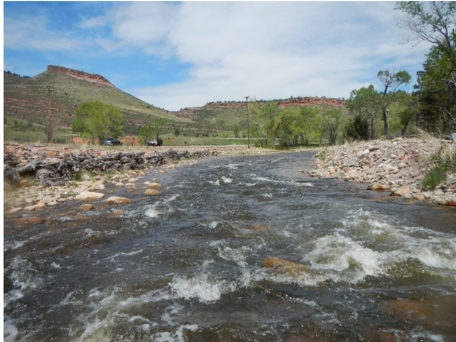
Figure 16. Existing Rootwad Protection at Hwy 7
