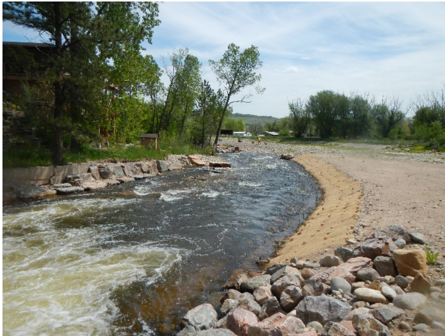
Figure 19. Longmont Diversion Post-Flood Work
