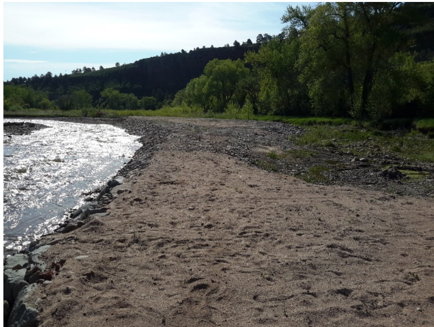
Figure 15. Post Flood Work at the "Plug"
