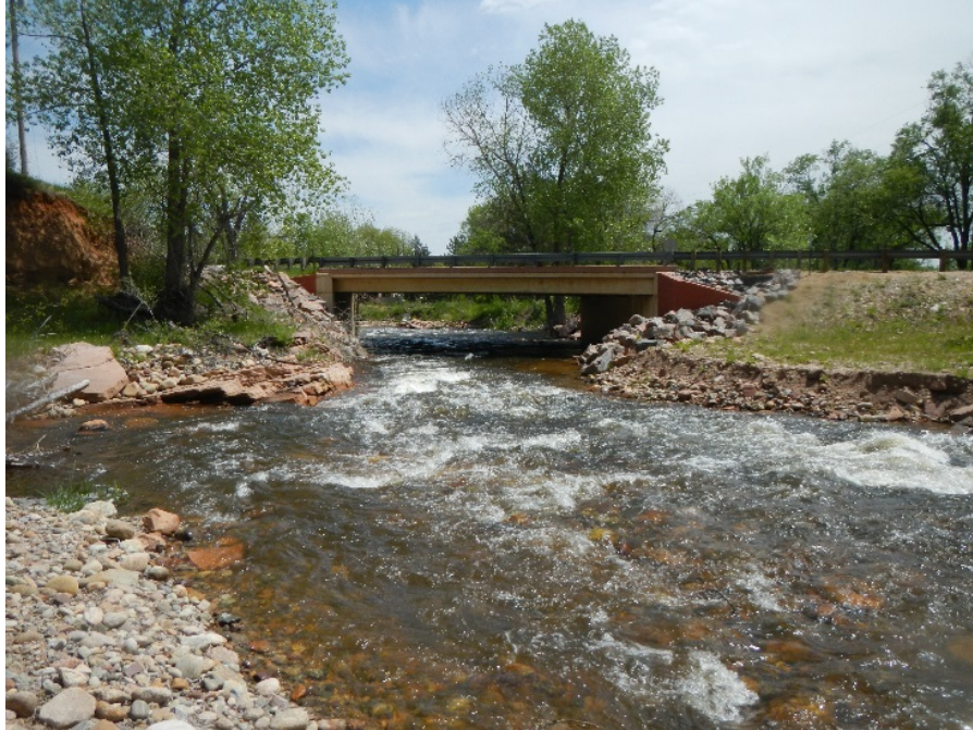
Figure 20. Downstream Extents of Project
