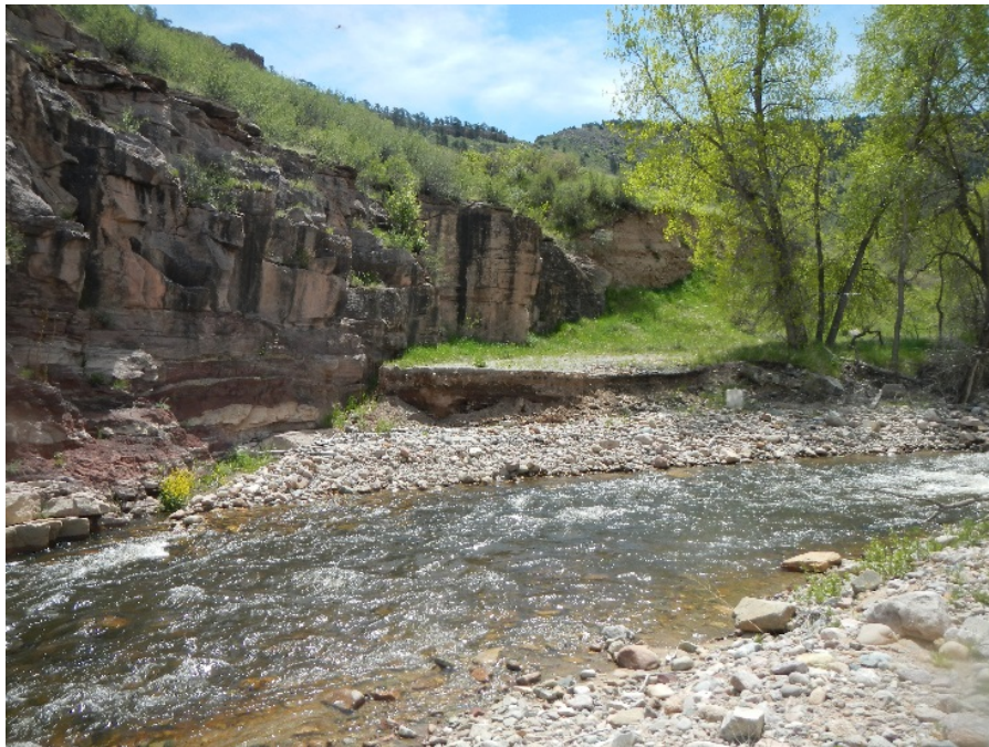
Figure 13. Damaged Old St. Vrain Road
