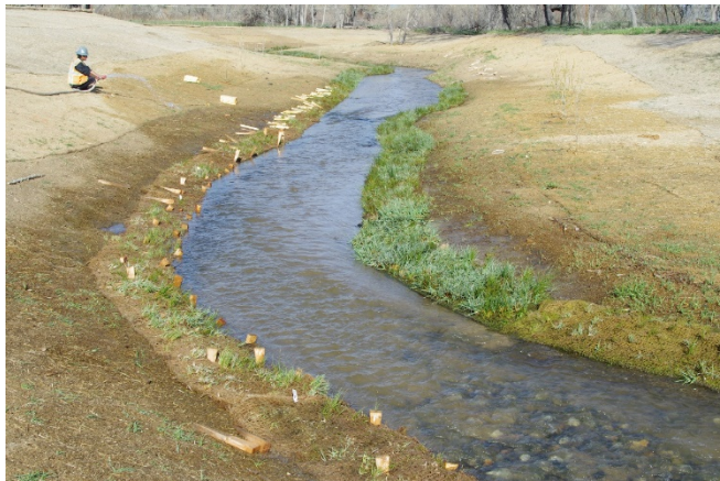
Figure 44. Wetland/Riparian Sod during installation: May 2016
