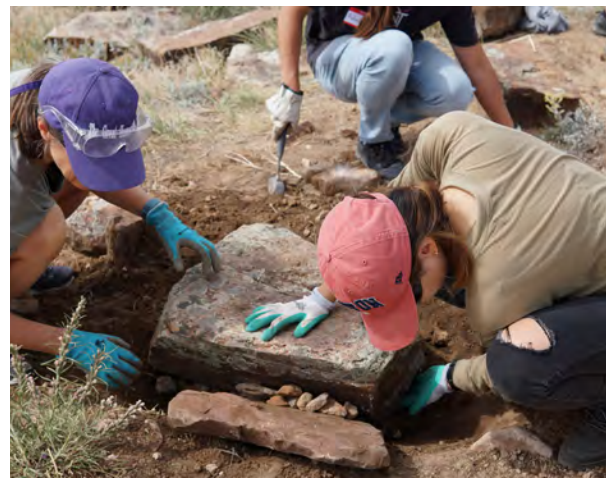
Volunteers placing stones to reduce trail width
