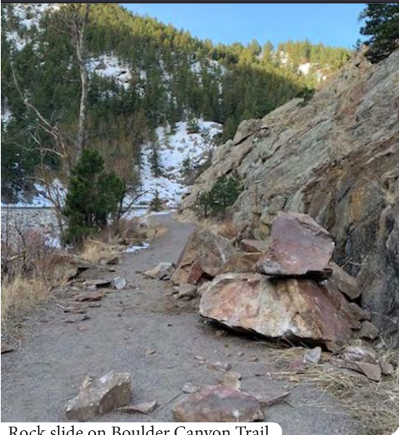
Rock slide on Boulder Canyon Trail
