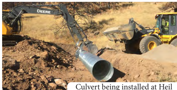
Culvert being installed at Heil
