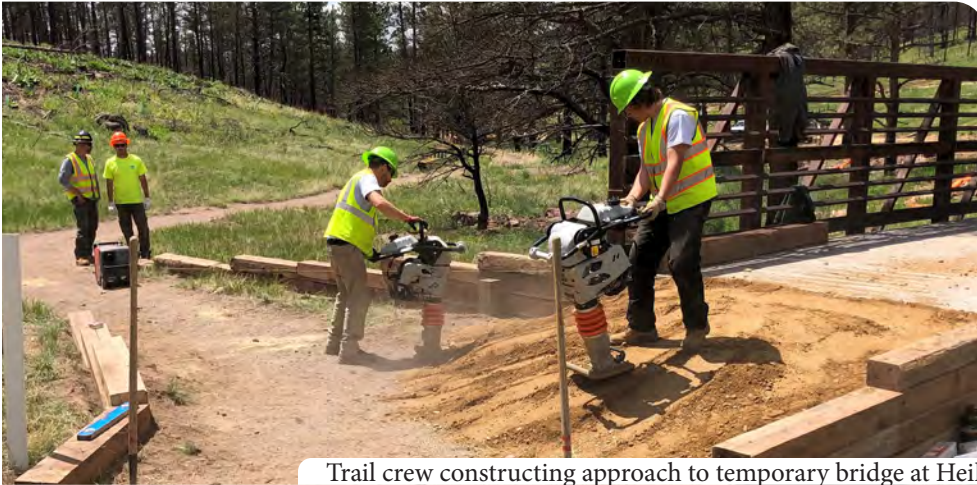
Trail crew constructing approach to temporary bridge at Heil
