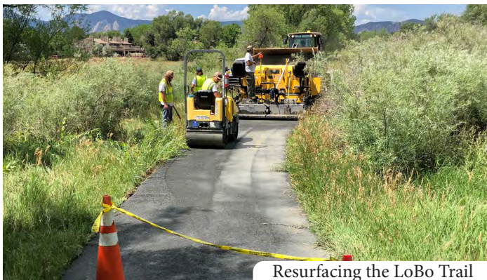
Resurfacing the LoBo Trail
