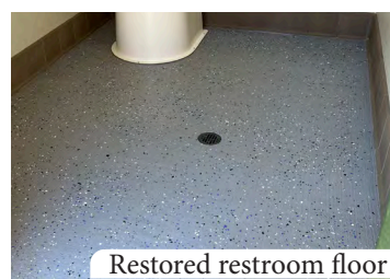
Restored restroom floor
