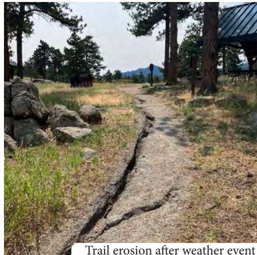
Trail erosion after weather event
