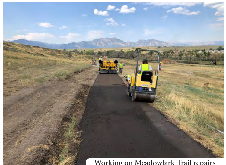
Working on Meadowlark Trail repairs
