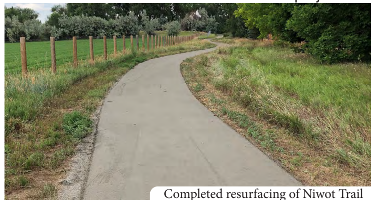
Completed resurfacing of Niwot Trail
