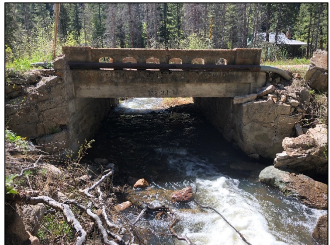
Figure B: Elevation view of upstream side
