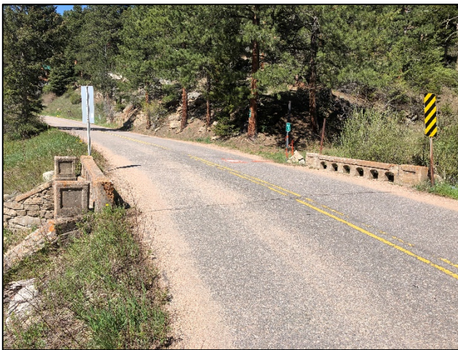
Figure A: General view Riverside Drive over Cave Creek
