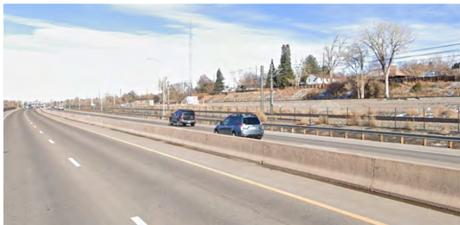
Figure 4. Example of a Cast-In-Place Concrete Barrier (US 85 (Santa Fe) between Aspen Grove and Sumner)
