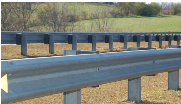
Figure 5. Example of a Metal-Beam Guard Rail Barrier
