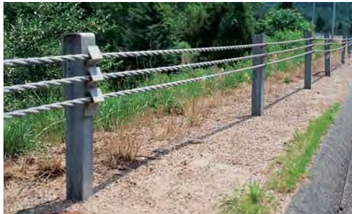
Figure 3. Example of a Cable Rail Barrier
