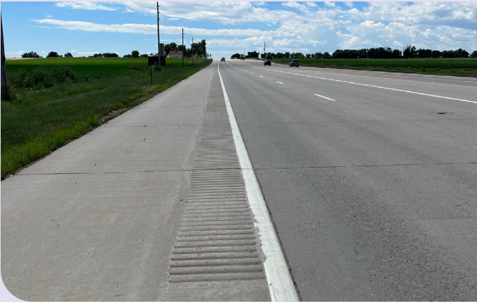
US 287 has edgeline rumble strips.
