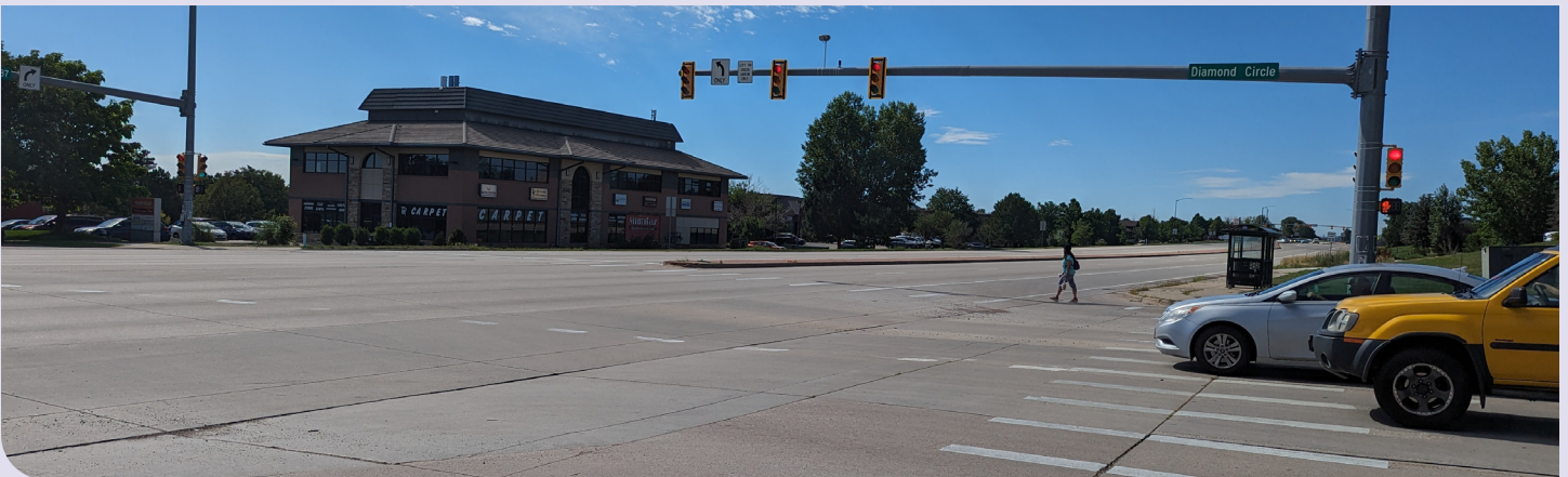
US 287 has long pedestrian crossing distances which increases pedestrian vulnerability.
