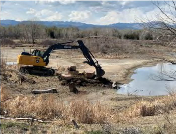
An excavator building the southeast fishing deck.
