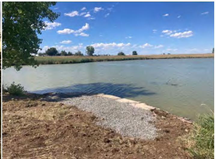
The West fish decks of Stearns Lake after construction was completed.
