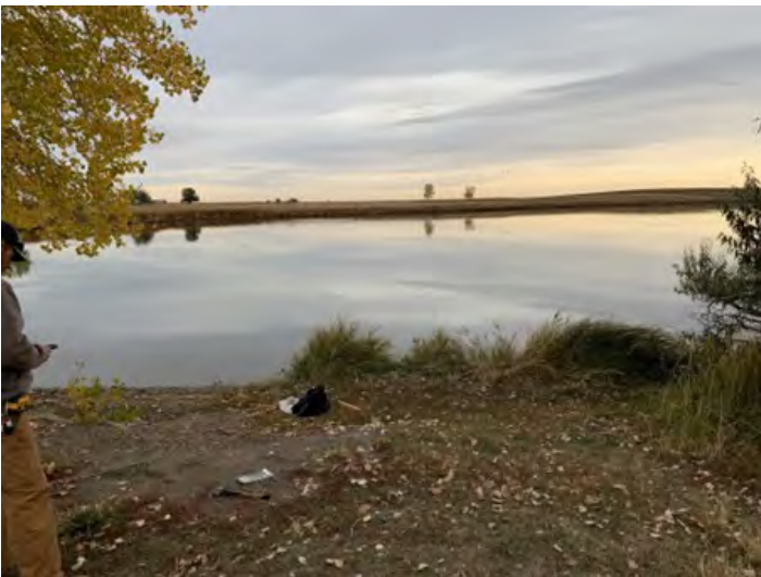
The West deck at Stearns Lake prior to building the platforms.
