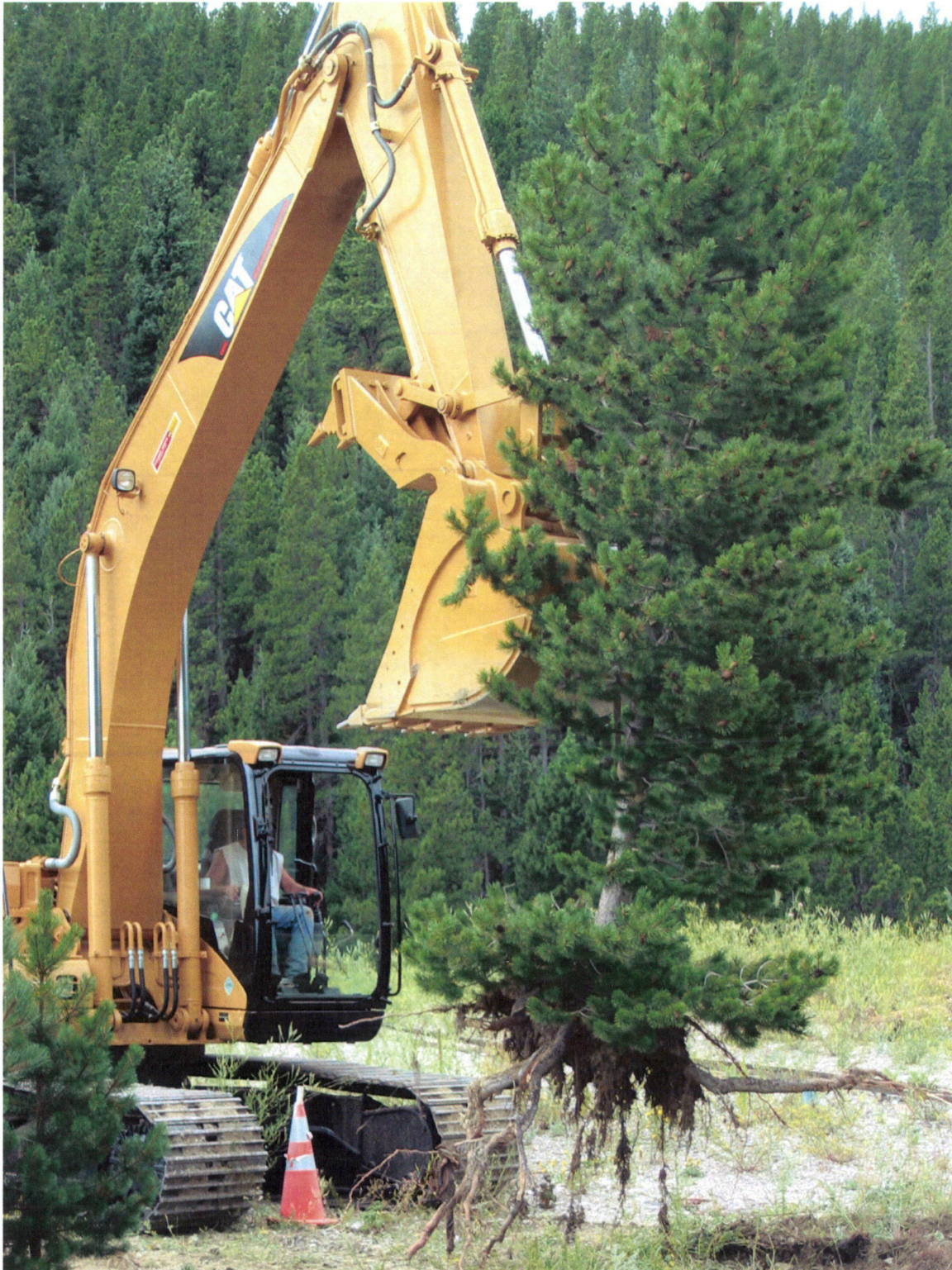
The site was initially cleaned and grubbed, beginning in August 2005
