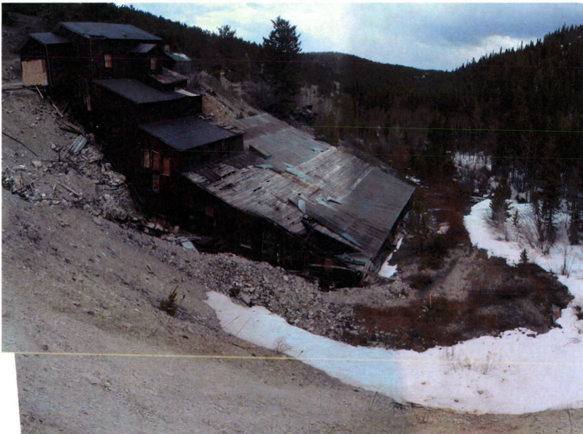
New Cardinal Mill building pre construction
