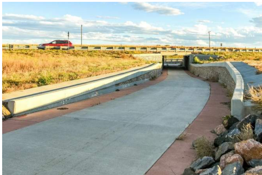
Airport Road Underpass
