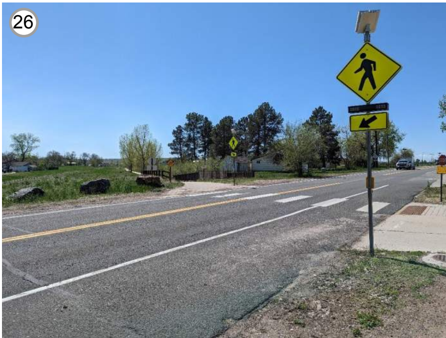
RTD ROW at East County Line Rd
