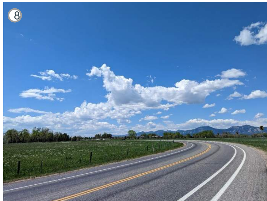
Valmont between 75 th and East Boulder – White Rocks Trail
