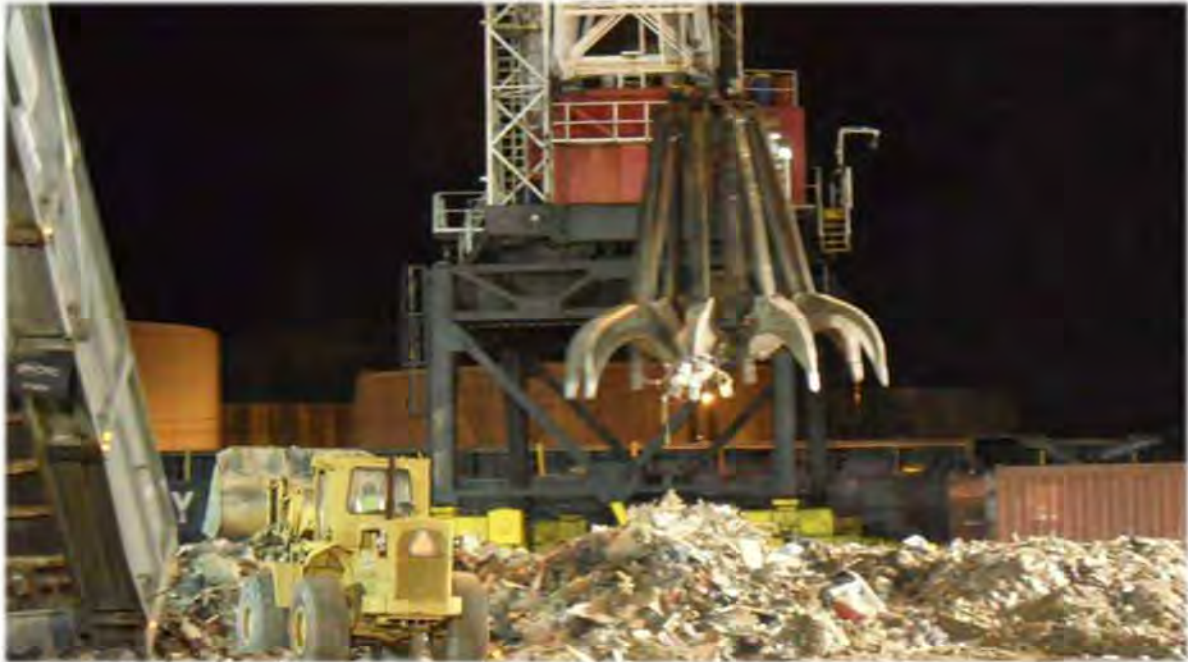
C&D Barging Site
