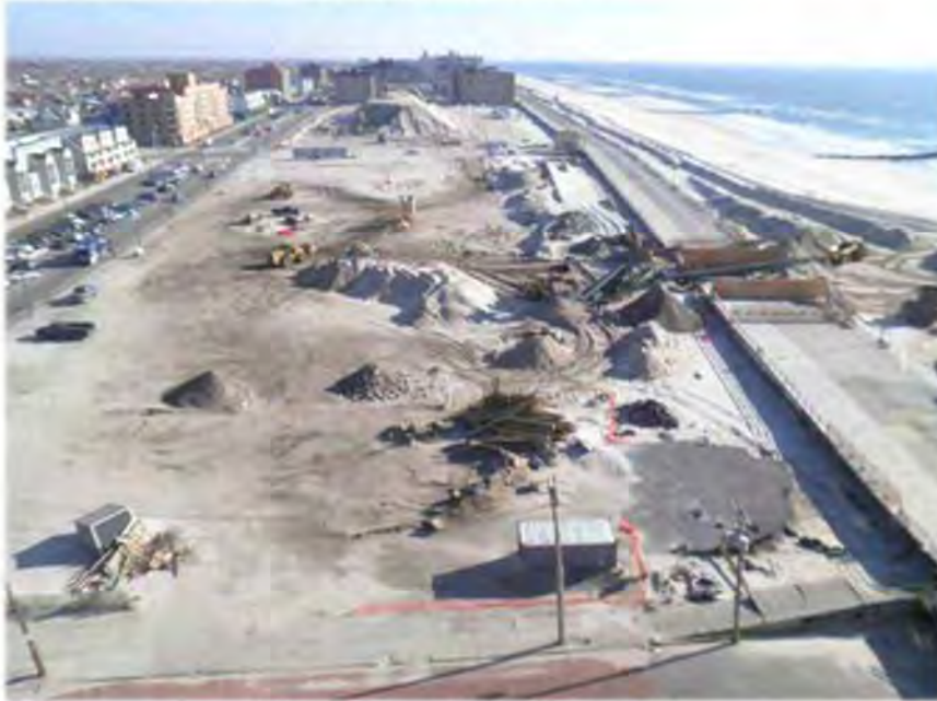
Sand Reclamation and Screening Site
