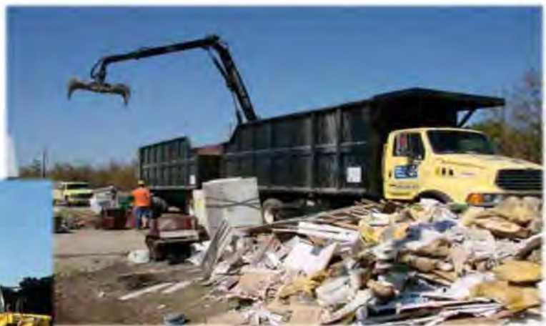
Curbside Pick Up C&D
