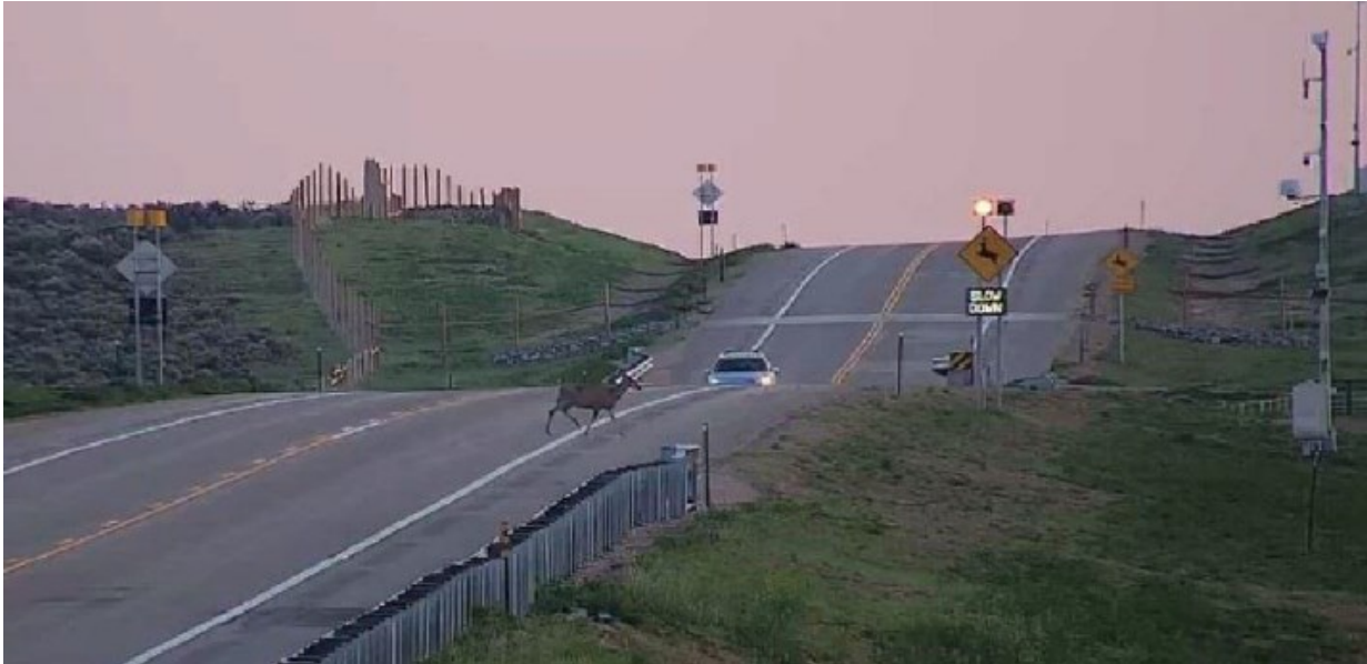
Photo 5. Example of a Wildlife Detection Zone
