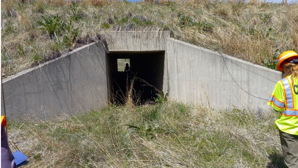
Photo D-14. Milepost 25.5
