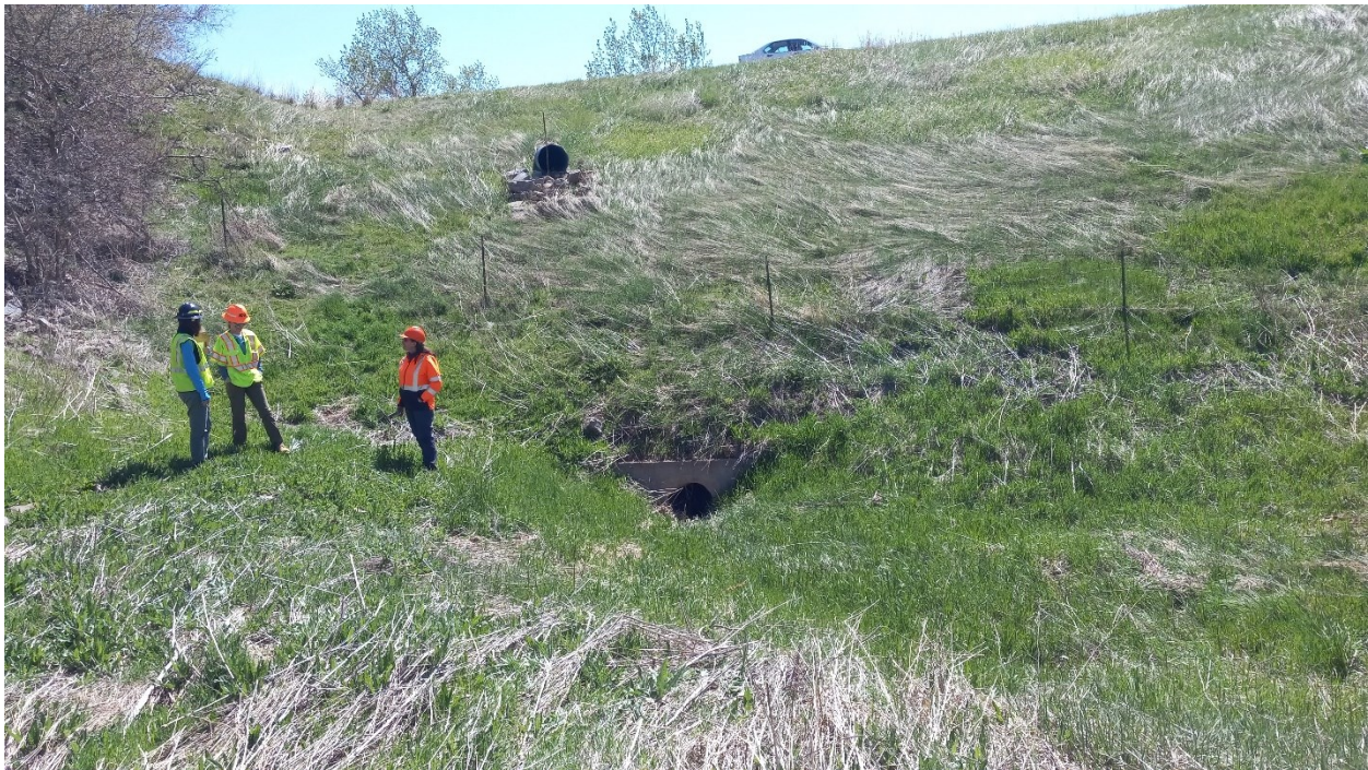
Photo D-13. Milepost 25.0
