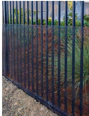
Example of a Herptile Barrier
