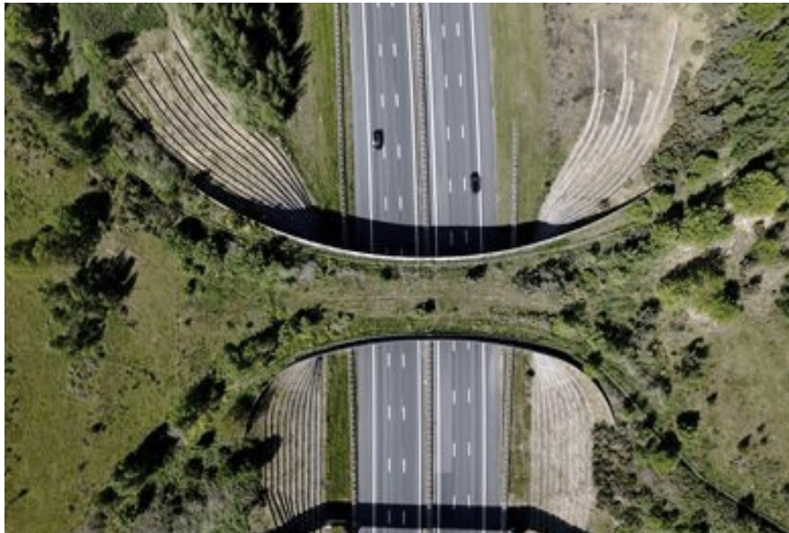
Photo 6. Example of hourglass-shaped overpass
