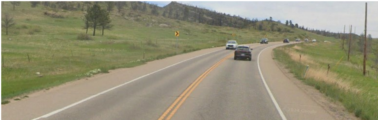
Photo 1. View of US 36 near MP 25.5
