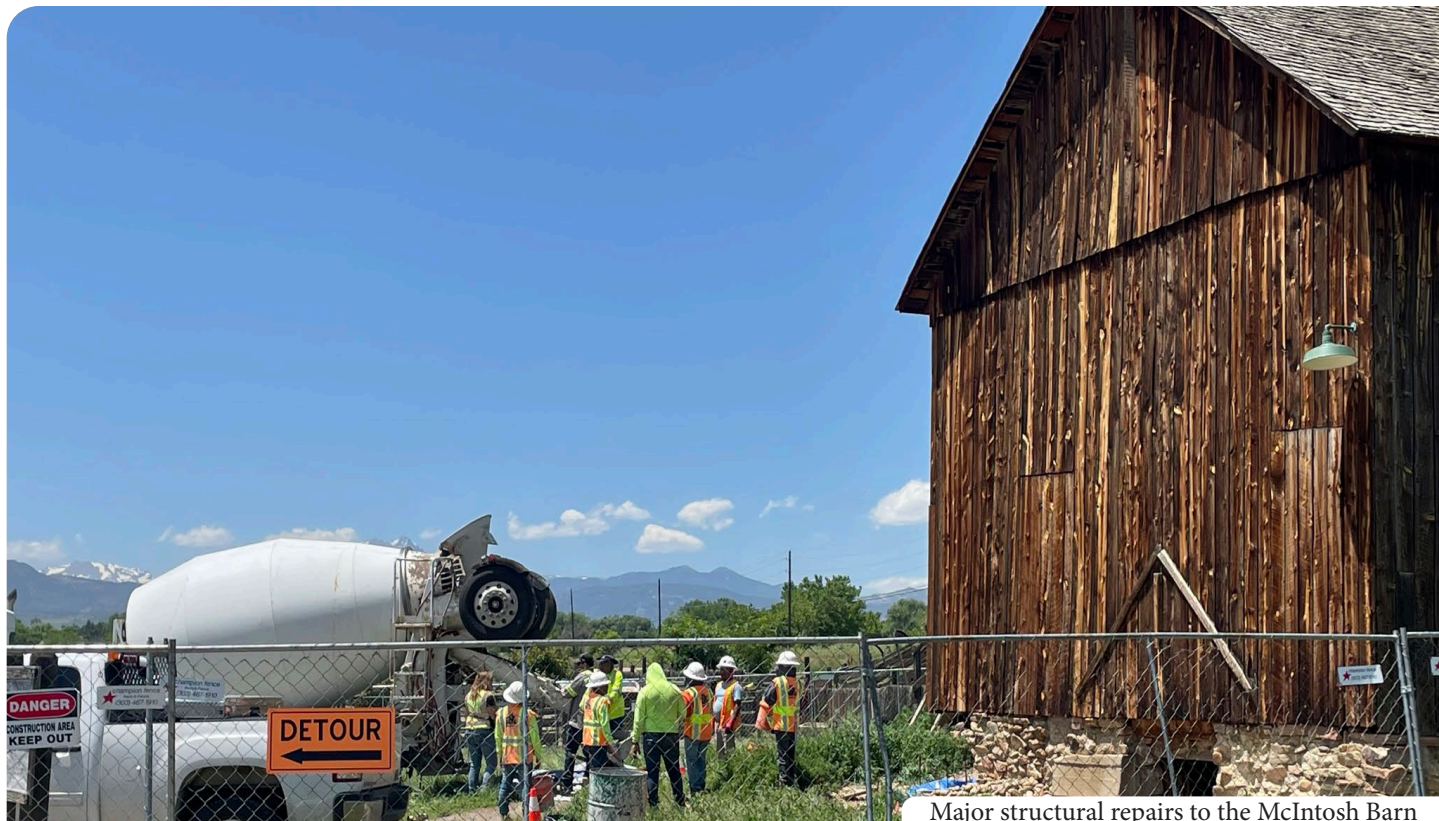
Major structural repairs to the McIntosh Barn
