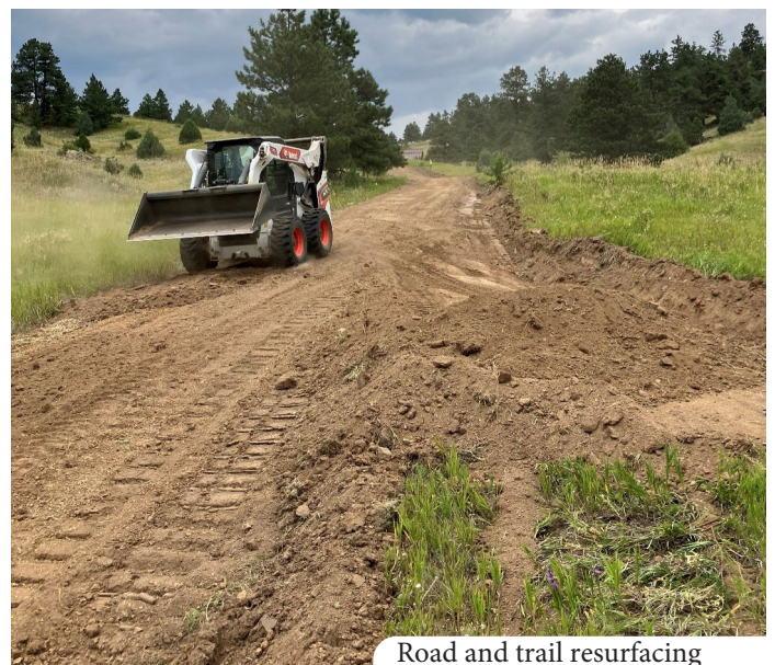
Walker Ranch Loop access road improvement
