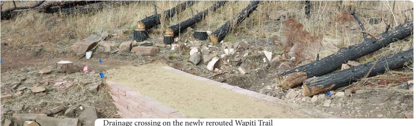
Drainage crossing on the newly rerouted Wapiti Trail
