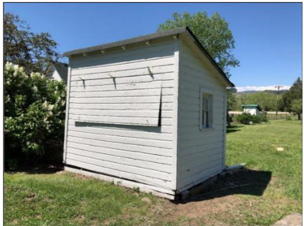
Figure 5. Northeast corner of the shed, facing southwest.
