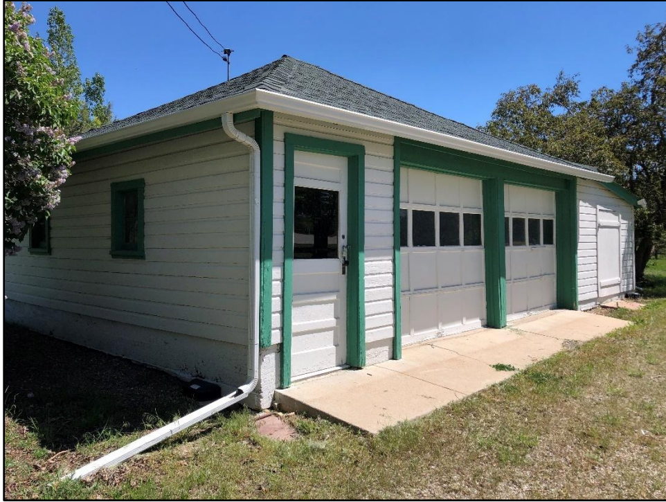
Figure 22. Southwest corner of the garage, facing northeast.
