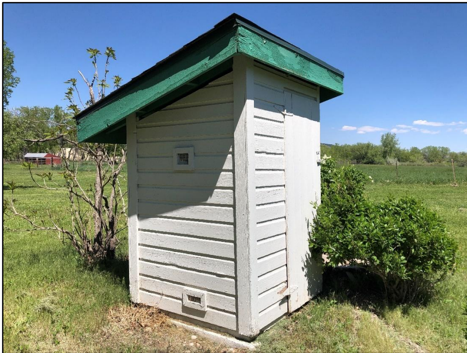
Figure 21. Southeast corner of the privy, facing northwest.
