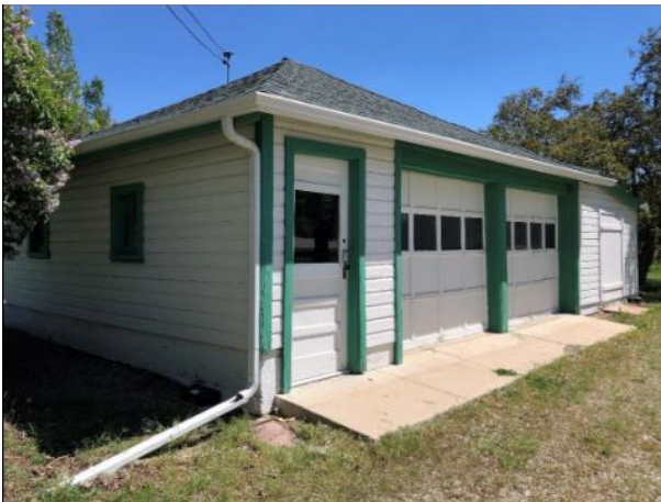
Figure 4. Southwest corner of the garage, facing northeast.
