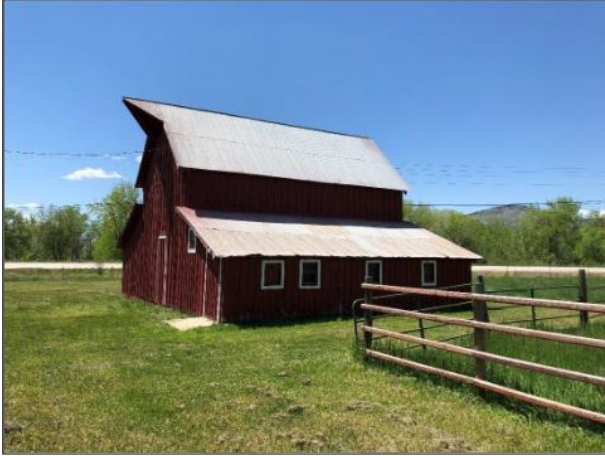
Figure 8. Northeast corner of barn, facing southwest.
