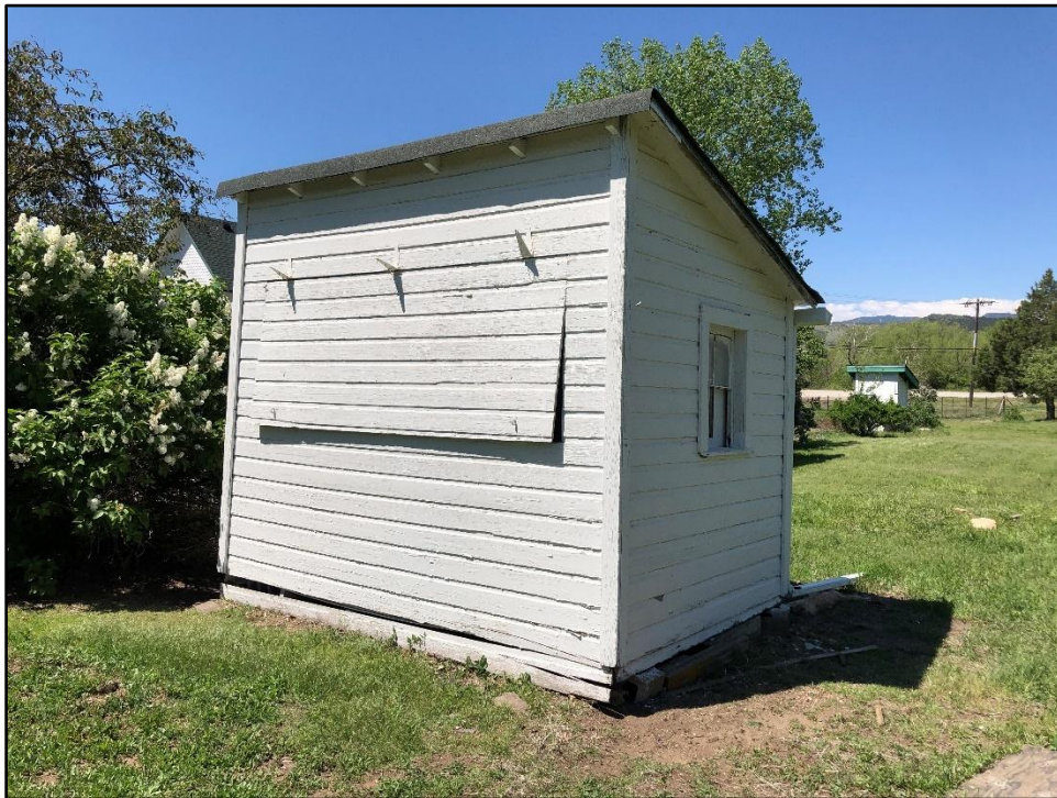
Figure 23. Northeast corner of the shed, facing southwest.
