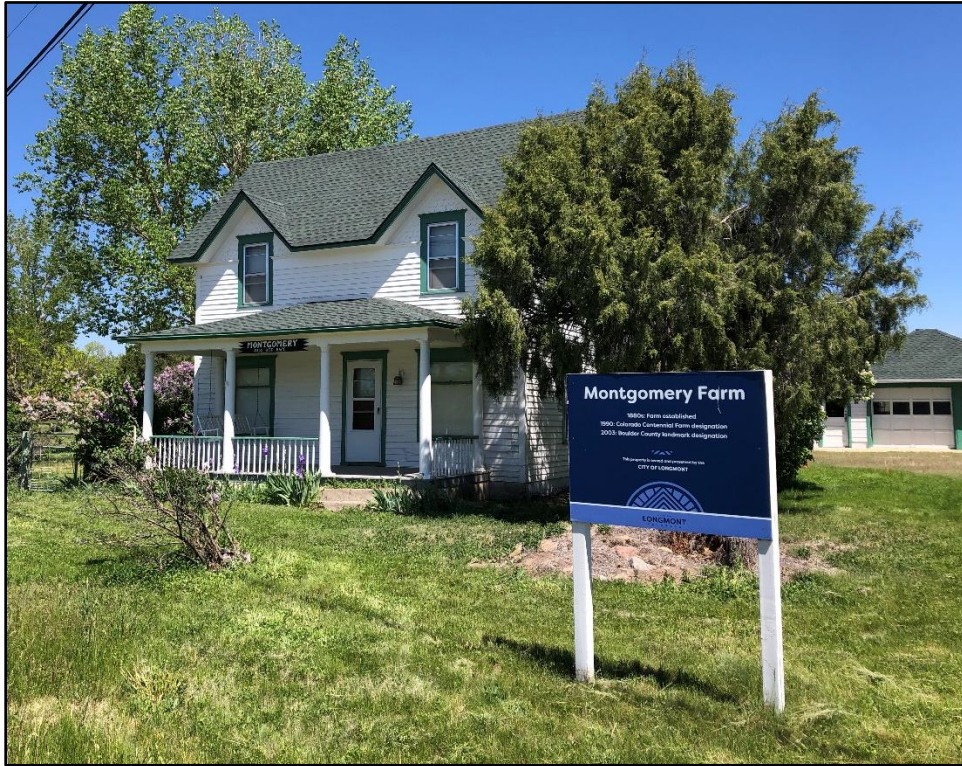
Figure 18. 5BL.4248 Montgomery Farmhouse, south facade.
