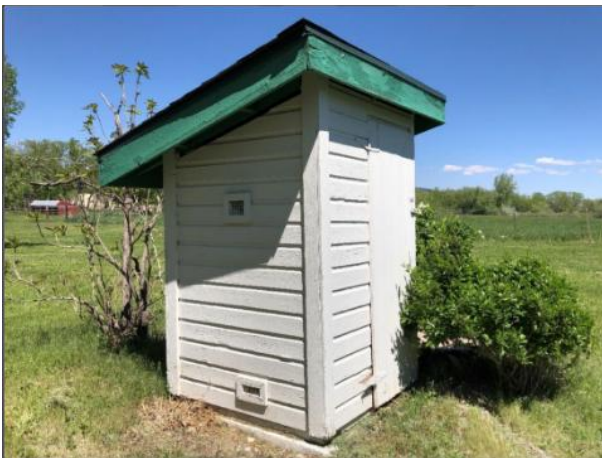
Figure 6. Southeast corner of the privy, facing northwest.
