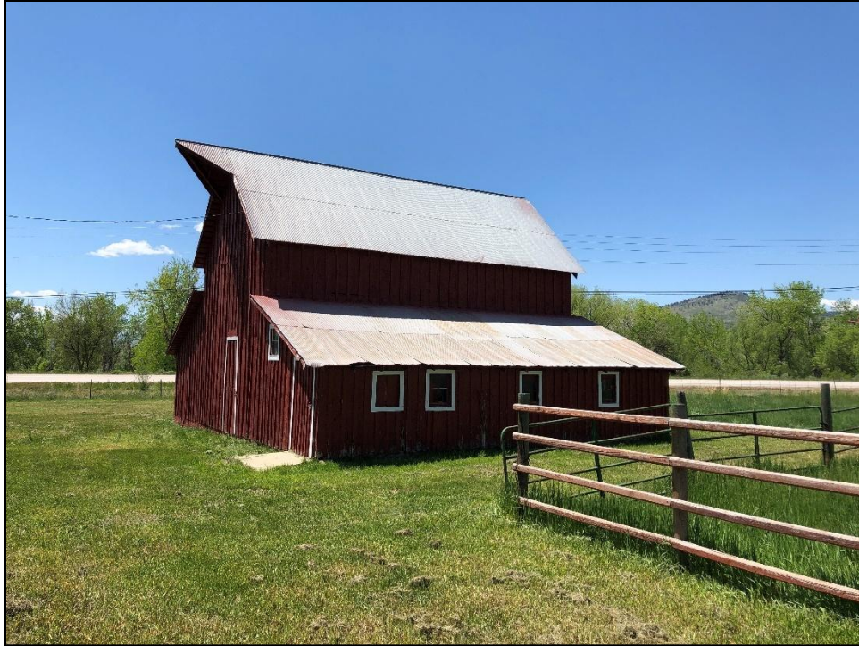
Figure 20. Northeast corner of barn, facing southwest.
