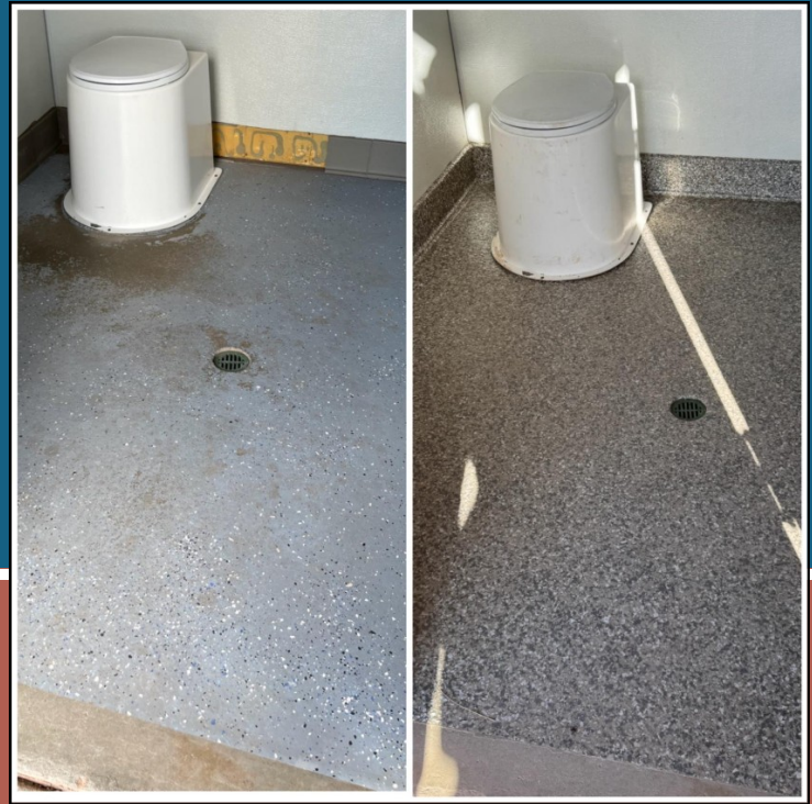
Pit toilet floor refinishing – before and after
