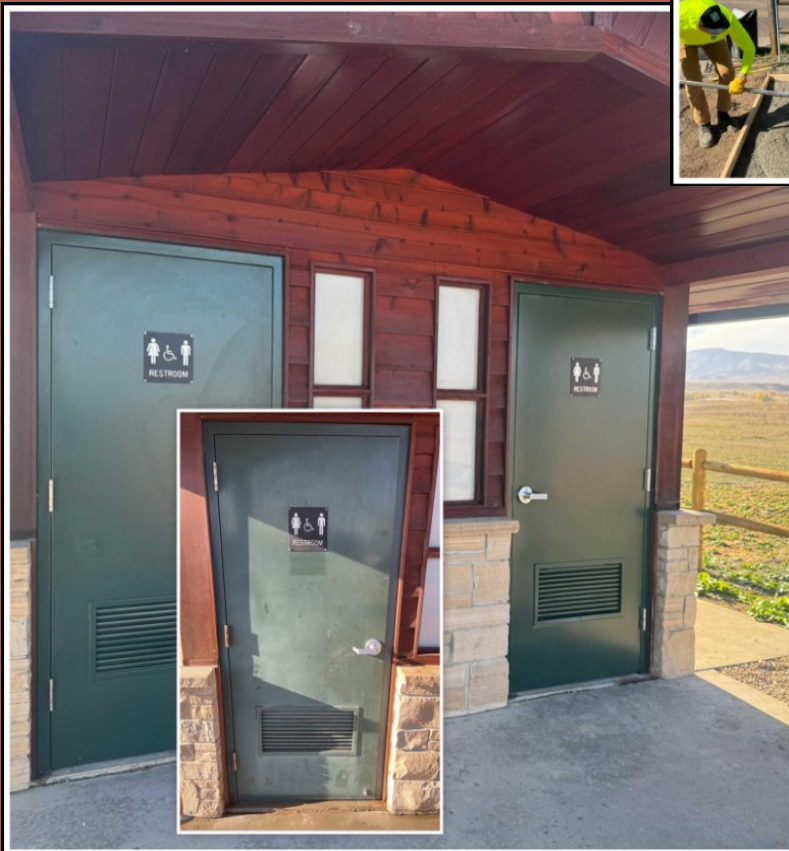
Lagerman Trailhead bathroom – before and after
