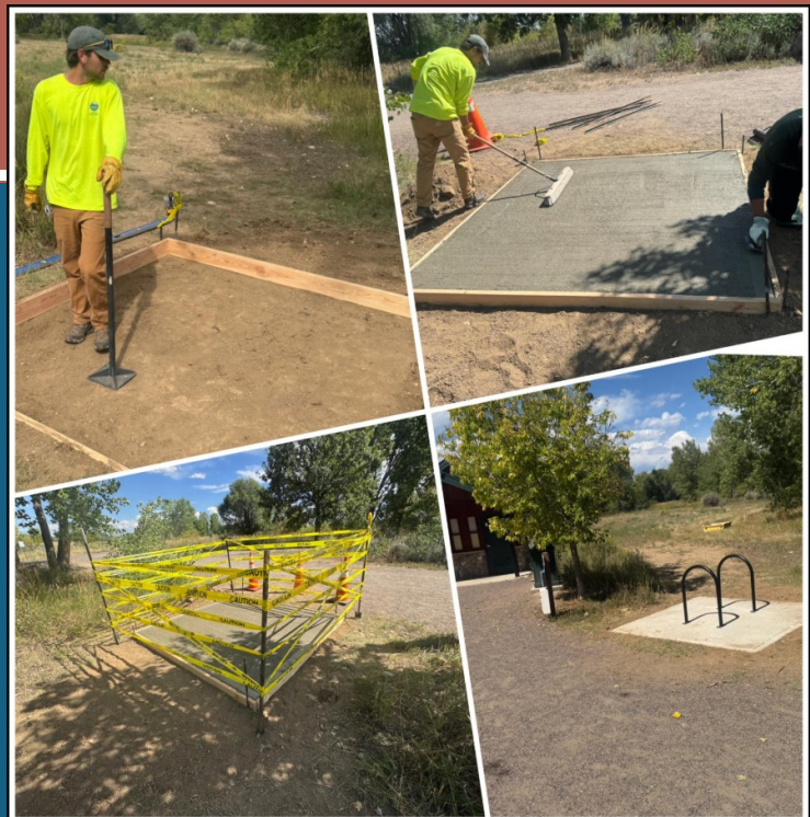
Installing a new bike rack at Pella trailhead
