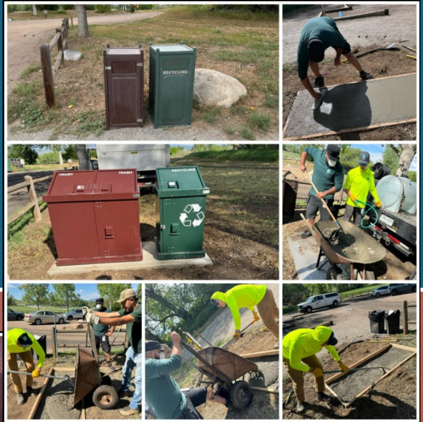
Bear Saver install at Niwot Loop Trailhead
